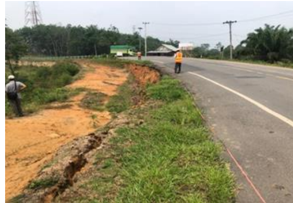
Fig. 6 Large displacement at MSE Wall
