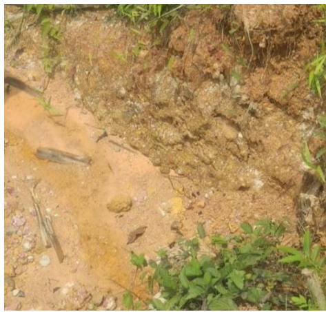
Fig. 9 Visualization of tuff material at toe of embankment
