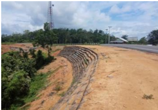
Fig. 5 Finished construction of MSE Wall
