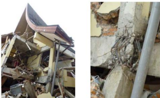
Fig. 1 A collapsed building and its damaged exterior beam-column joint [2].
