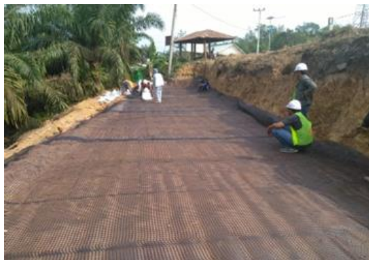
Fig. 3 Soil reinforcement using uniaxial geogrid
