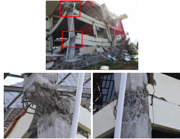
Fig. 9 A collapsed building due to the 2018 Palu Earthquake and damage to the exterior beam-column joints. (Photo courtesy of Syafri Wardi)
