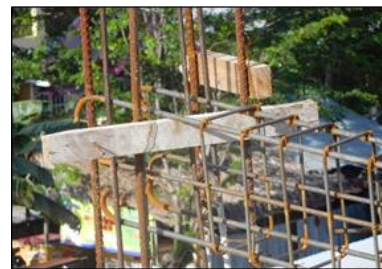
Fig. 2 Substandard detail of exterior beam-column joint in construction [4].
