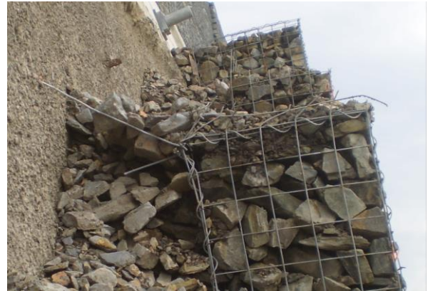
Fig. 2 Detail of steel wire attachment partially unfolded during usage
