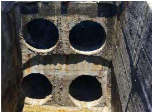
Fig. 2 Culverts serving as caisson breakwaters in connection with the ocean and the harbor
