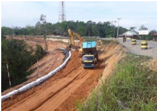
Fig. 4 Compaction of embankment above soil reinforcement
