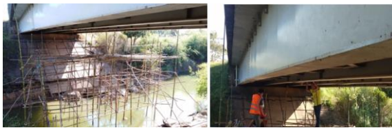
Fig. 10 Installation testing instruments for Brg. No.11.
