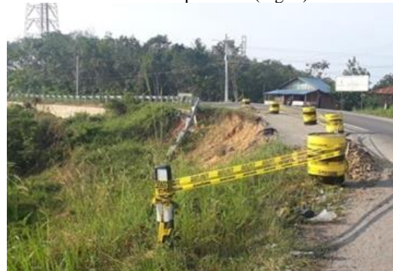
Fig. 1 Slope surface instability due to water runoff
