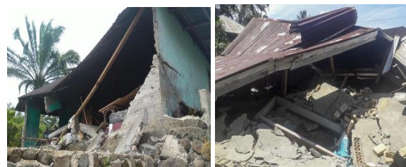
Fig. 1 Damage to brick wall houses due to the 2022 West Pasaman earthquake [5].
