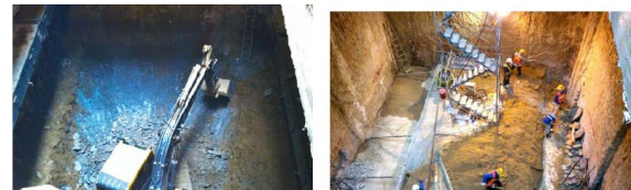
Fig. 5 Final excavation base at a depth of 32.5 m for IDT shaft
