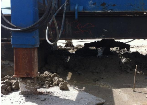
Fig.5 DMM installation.
