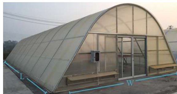
Fig.1 Large sized parabolic greenhouse solar dryer.
