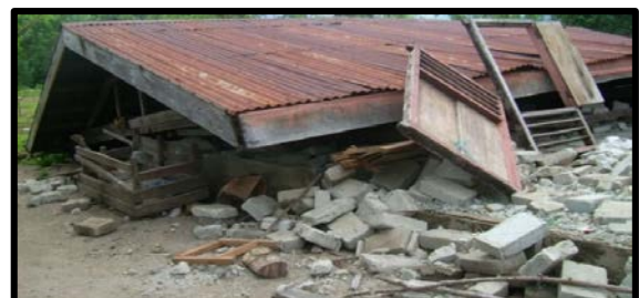
Fig. 2 Collapse of a hollow brick building [3]
