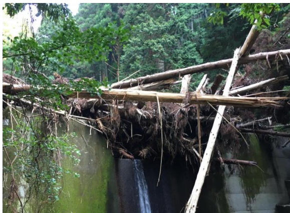
Fig. 13 Woody debris trapped at the sabo dam.
