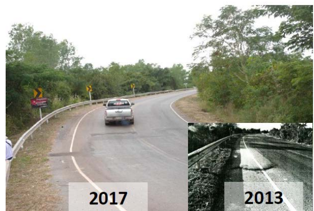
Fig. 14 crack due to horizontal movement
