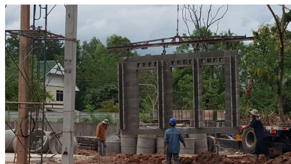
Figure 1. The rapid construction of wall using preformed concrete blocks
