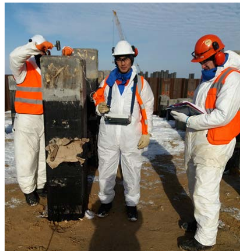
Fig.1 Procedure pile foundations of PIT on construction site “Prorva”.
