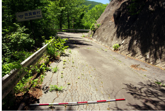
Fig. 4 Deterioration of road surface in the closed section of Gonbei Highway Cracks, accumulated fallen leaves, and scattered invading weeds can be observed. Length of the red and white striped pole = 2 m.
