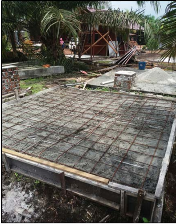
Fig. 2 Reinforcement of concrete slab before casting concrete slab
