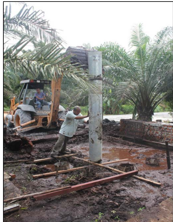
Fig. 1 Adjusting pile verticality during piling
