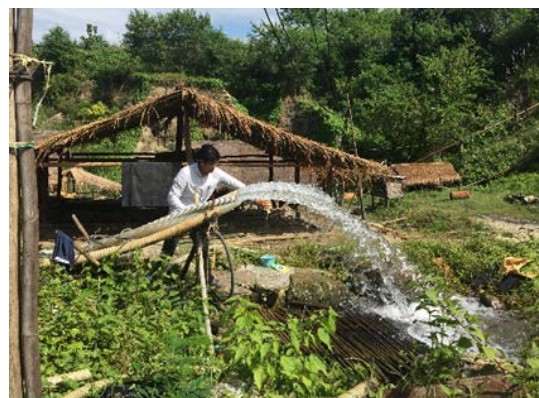
Fig. 2 Groundwater leaked form the tunnel
