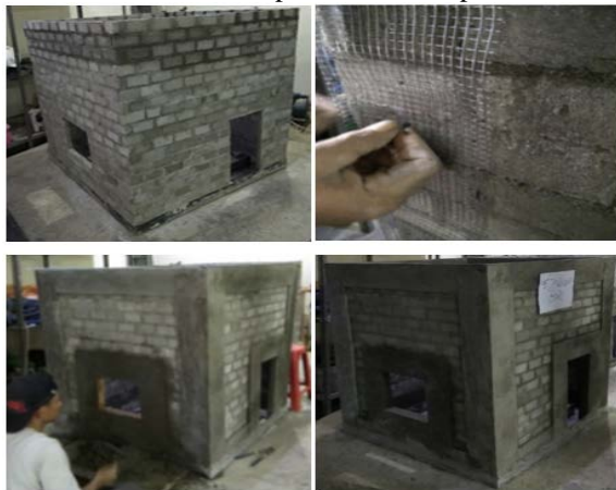
Fig. 5 Construction Process of the Specimens B1 and B2
