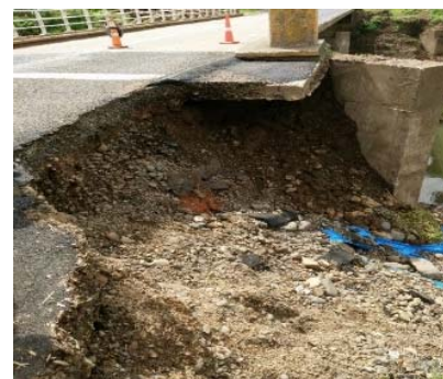
Fig.8 Erosion of soil under the road near the bridge abutment at site F
