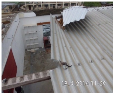
Figure 3. Failure of roof cladding
