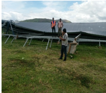
Figure 8. Collapse of steel structure
