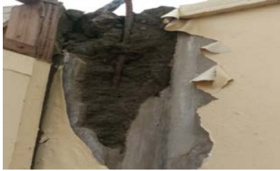
Figure.12 Failure of wall due to use of river gravel
