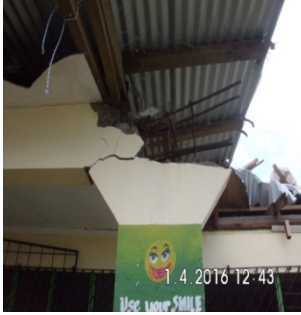
Figure 7. Column beam joint failure
