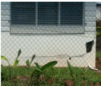
Figure 9. Masonry wall failure
