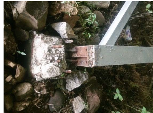
Fig.12 Foundation failure at site H
