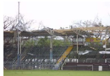
Figure 2. Complete damage of roof of the stadium Figure 2 shows the complete destruction of roof
