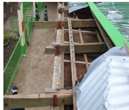
Figure 5. Roof members made with boxing timber
