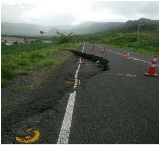
Fig.13 Road failure at site I
