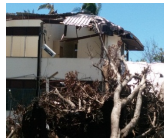
Figure1. Damage of roof due to fallen tree
