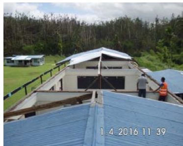
Figure 4. Failure of roof and roof truss
