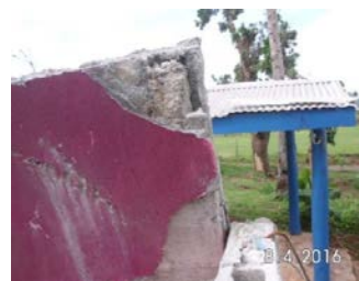
Figure 11. Failure of wall due to lack of Corner block and reinforcement binding
