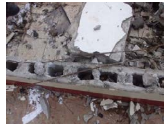
Figure 10. Wall failure due to poor workmanship
