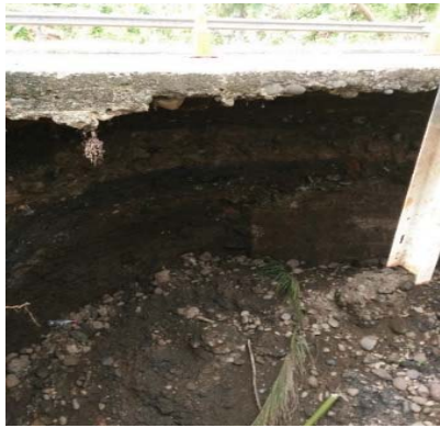
Fig.9 Sinkhole formation alongside the road over the creek at site G.
