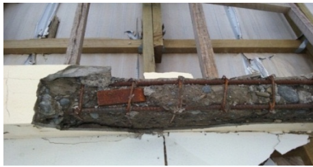
Figure 13. Beam with insufficient cover and poor quality materials
