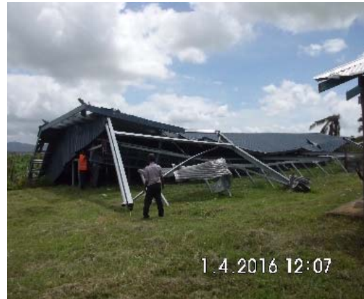
Fig.11 Failure of steel structure at site H
