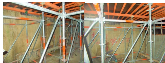
Fig. 12 Photo of B3 after removal of bracing layer 2.
