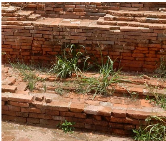
Fig.1 Deterioration of the restorative brick (Photograph taken in August 2014)
