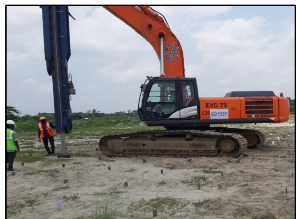
Fig. 5 Installation of Prefabricated Vertical Drain
