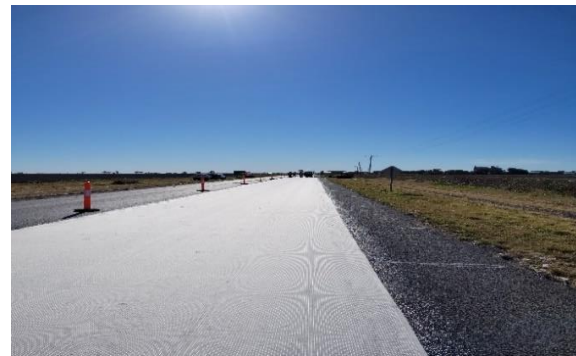
Figure 4: Geotextile on tack coat
