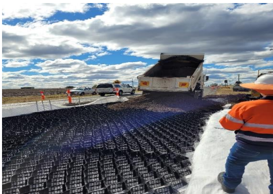
Figure 7: Placing material and fill voids
