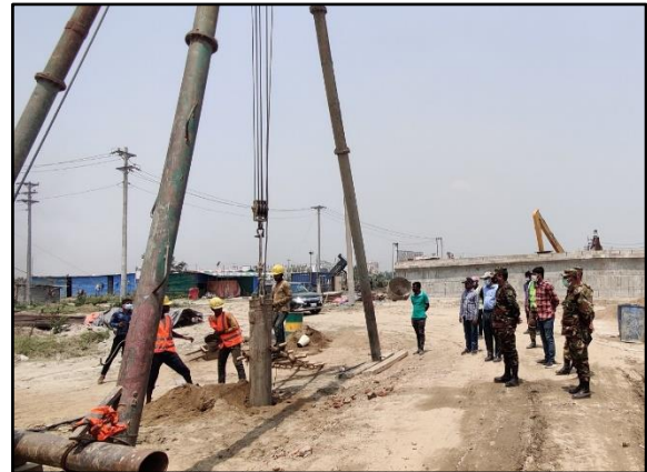
Fig. 4 Sand Compaction Pile (SCP) installation
