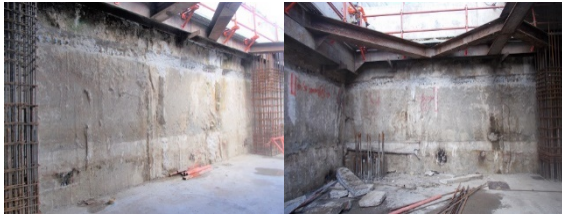
Fig. 13 Photo of B2 after removal of bracing layer 2.
