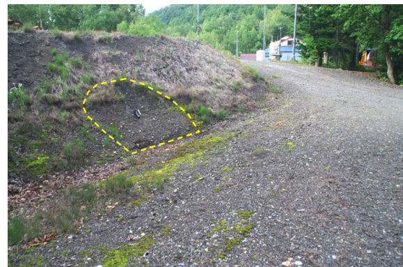
Fig.1 Protecting ground surface by RAP
