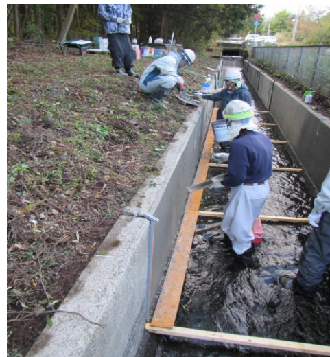
Fig.1 workers repairing a deteriorated river canal in Kochi.
