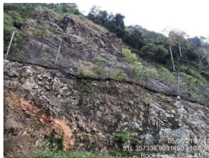
Fig. 3 Rockfall Net Fence KM18 Ende-Datusuko, Flores Indonesia
