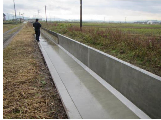
Fig. 2 A well repaired river canal repair in Kochi
