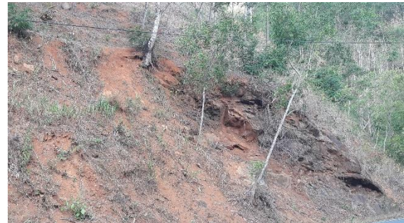
Figure 2: Slope failure on basaltic andesite rock with sheathing joint
