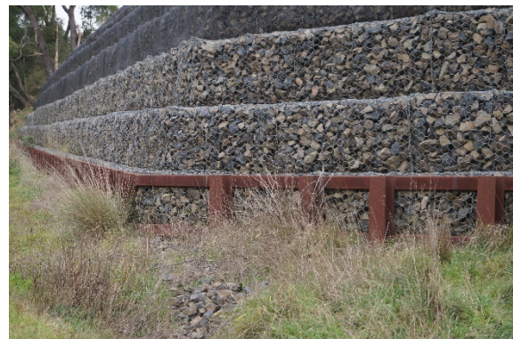
Fig. 1. GF-GR-RW with piles used in South Gippsland
