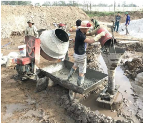
Fig. 3 CFG pile construction process
