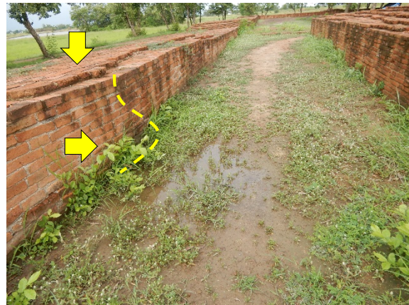
Fig. 5 Deformation of brick wall at Wat Krasai (Photograph taken on May 17, 2017)
