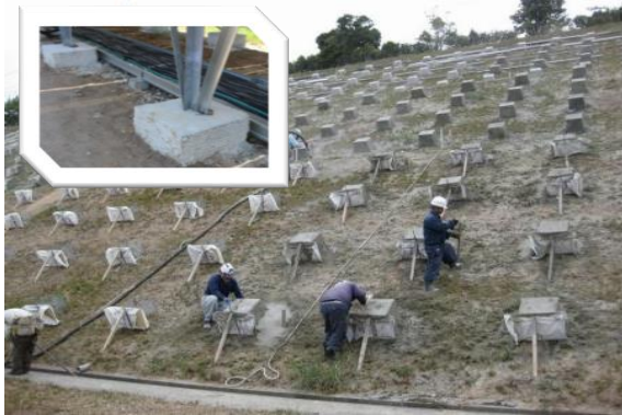
Fig 9 Sakura-no-Sato MPP, Casted mortar foundations with steel mounting frame attachments (source: Toda Corp, Nikkei B.P.)
