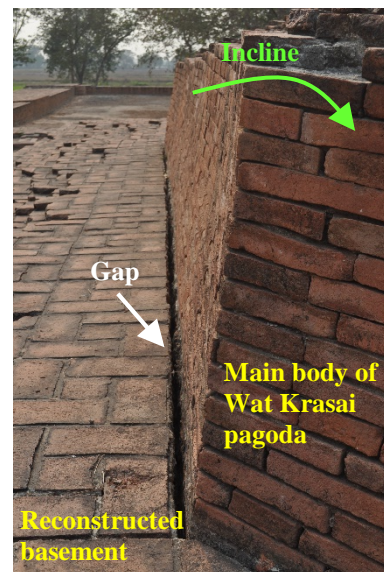
Fig. 6 The gap between the main body and reconstructed basement of the pagoda (Photograph taken on August 20, 2019)
