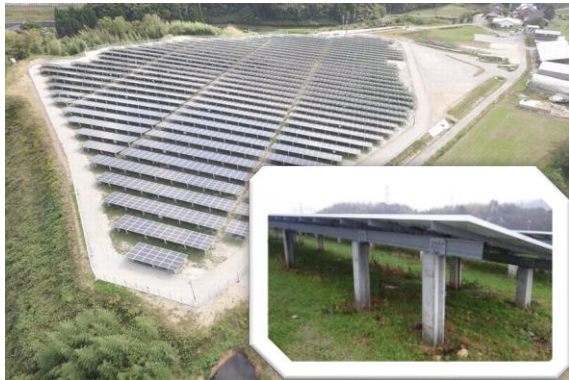
Fig. 6 Exeo Matsue Solar Farm H Pile foundations assembly (source: Kyowa Exeo)
