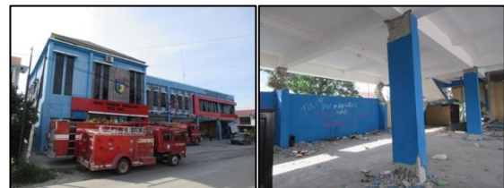
b). The Fire Station building and damaged columns
