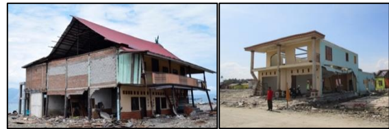
Photo 1 Damage on confined masonry structures
