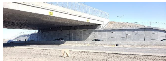
Fig. 1 South Abutment MSE Wall
