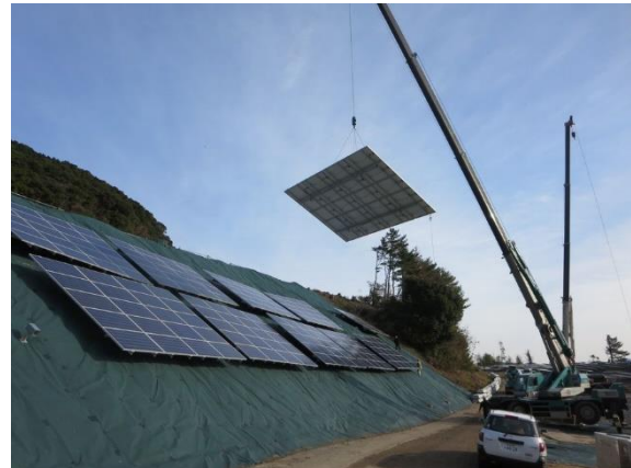
Fig.3: Installation of solar panels on side slopes. (Source: Daiwa Lease/Daiwa House Industry).
