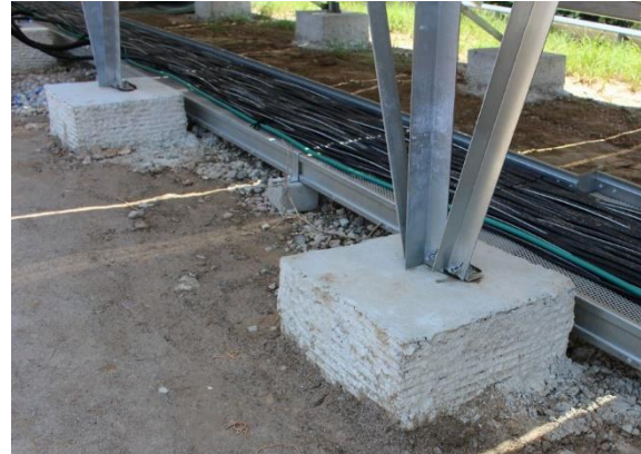
Fig.7: Foundation method of “spraying” mortar in a square mold with buried steel beams was used. (Source: Nikkei BP)
