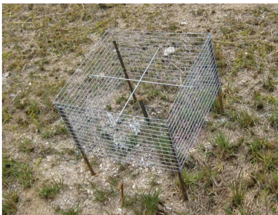
Figure 6: Foundation method using a net square mold. (Source: Toda Corp)
