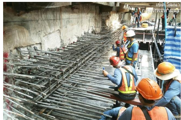
Fig. 8 Band beam during construction
