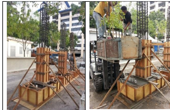
Fig. 4: Pouring of wet concrete into formwork on corner beam-column joints at construction site.
