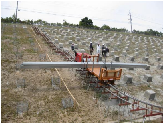
Fig.5: A monorail was constructed to transfer heavy materials. (Source: Toda Corp)
