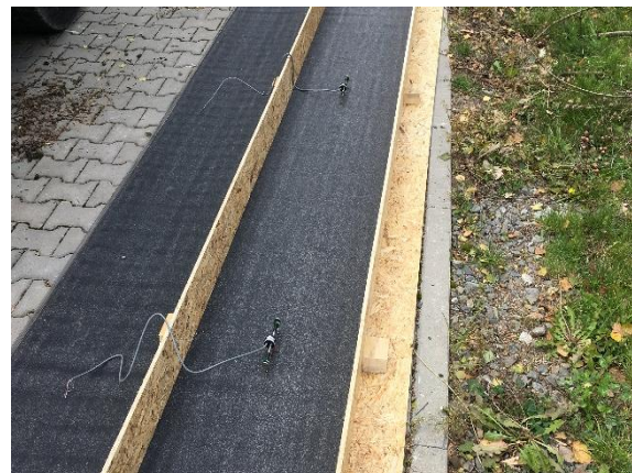
Fig. 1 Installation of string strain gauges
