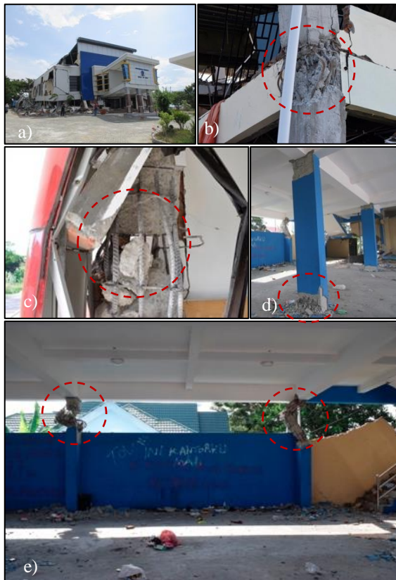
Photo 4 Typical damage of RC structures: a) The first story collapsed due to the soft story, b) Failure of beam-column joint, c) Shear failure of short columns, d) Shear failure of columns e) Buckling of longitudinal reinforcements of a column
