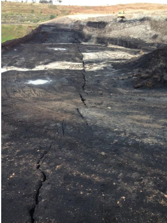
Fig. 4 Major cracks on North Batter in November 2013
