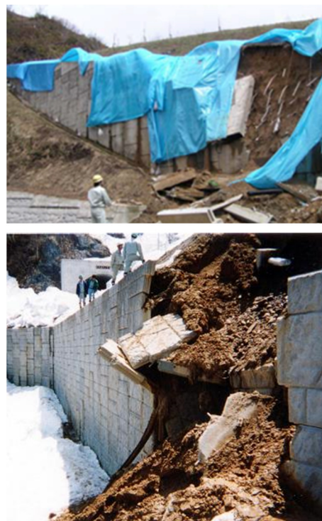
Photo 1 Deformation case of reinforced soil walls
