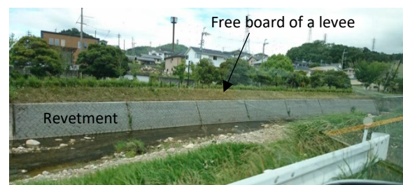
Fig. 4 Revetment and Free board of a levee
