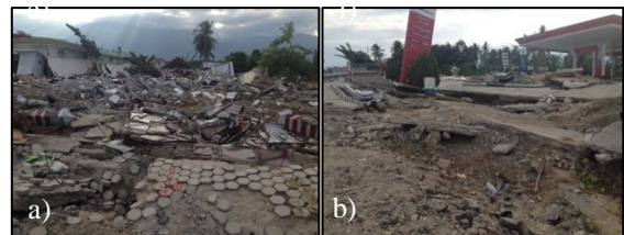
Photo 3 Damage due to liquefaction: a) Swept away homes, b) Damaged fuel station facility
