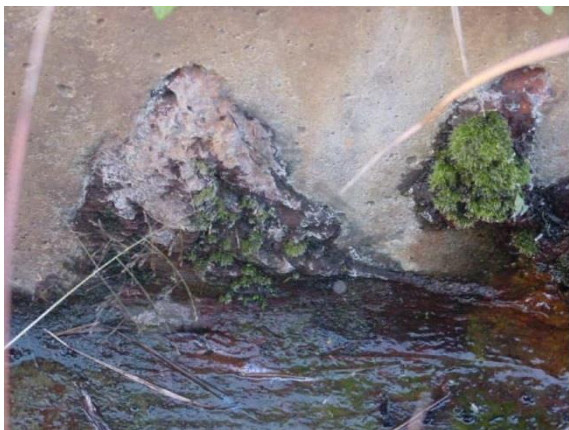
Pic. 4 Concrete deterioration by acid soil
