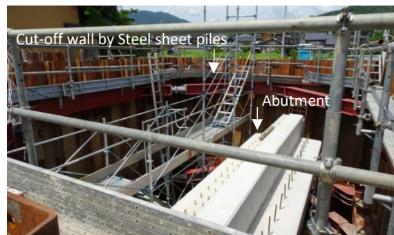
Fig. 2 Construction space by excluding water using steel sheet pile
