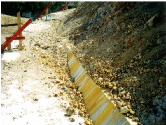
Pic. 5 Discoloration of concrete by acid soil
