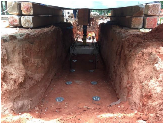
Fig. 7 Footplate Installation.
