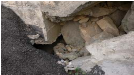
(b) Failure with cavity generation
