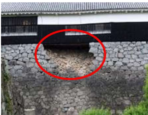
(b) Situation after the disaster Fig. 9 Failure the stonewall of H323
