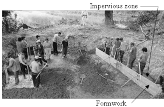
Fig. 6 Compaction of impervious zone by the wall making method
