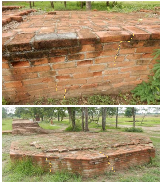
Photo 3 Cracks of brick structures
