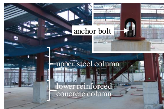
Photo 1 Practical application of proposed connection
