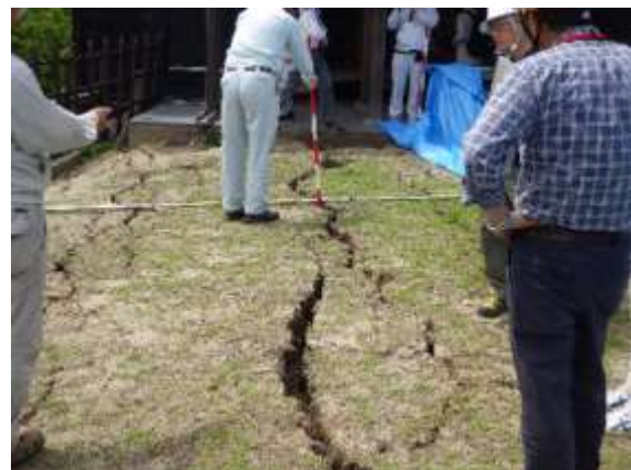
Photo 2 Cracking embankment
