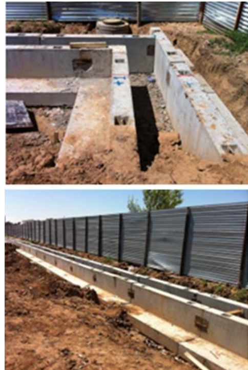
Fig. 8 Construction of guide wall in site ADP.
