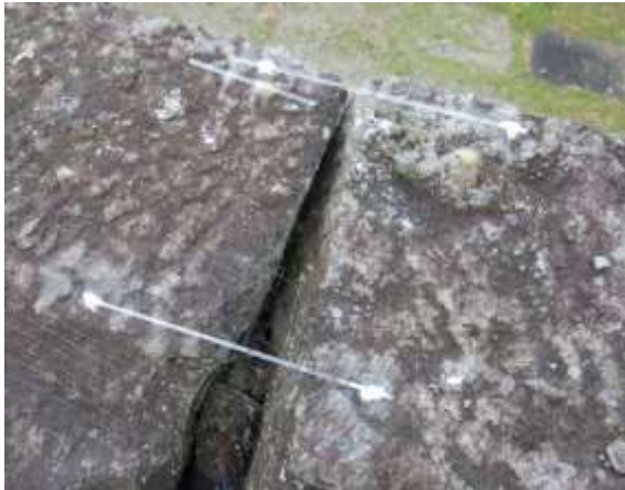
Photo 3 Glass rods for monitoring displacement between stones
