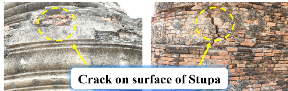
Fig. 1 Example image of cracks on the surface of stupas visible in many locations around Wat Chai Wattanaram, a temple located in the historic province of Ayutthaya, Thailand.
