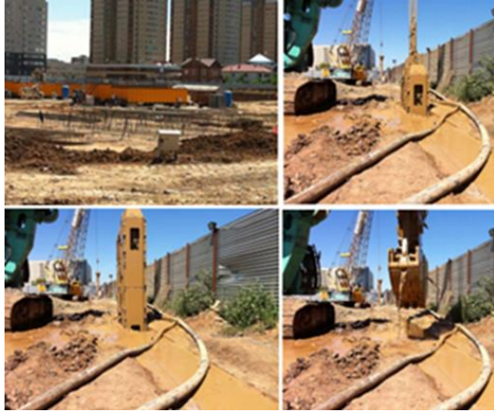
Fig. 9 Excavation for the diaphragm wall in ADP.
