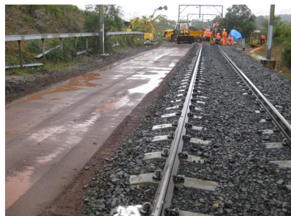
Fig. 1 Ballast and capping layer [2].
