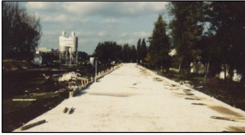
Fig. 1 Concrete raft used as a floating housing road in the Netherlands [13]
