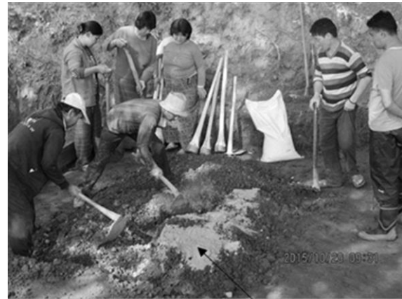
Fig.5 Stabilization treatment of foundation by cement-mixed soil
