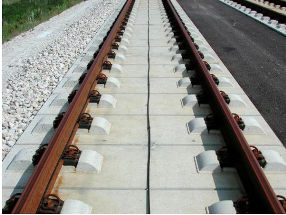
Fig. 1 A typical slab track
