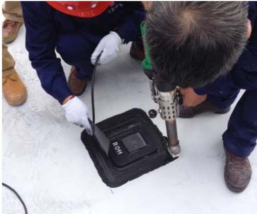
Fig. 11 Combi-Module embedded in Leak location liner.
