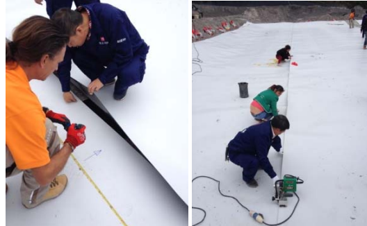
Fig. 8 Extra piece insert and welding in progress.
