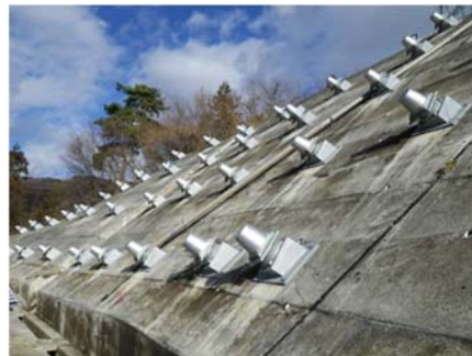
Figure 1 Ground anchors in a retaining wall.
