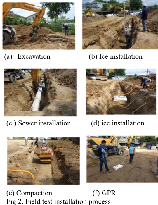
Fig 2. Field test installation process
