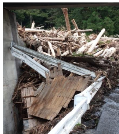
Fig. 10 Woody debris trapped the rail bridge
