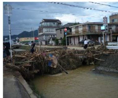
Figure 1 Log jam formation around the bridge (Sep. 2014, Fukuchiyama city)
