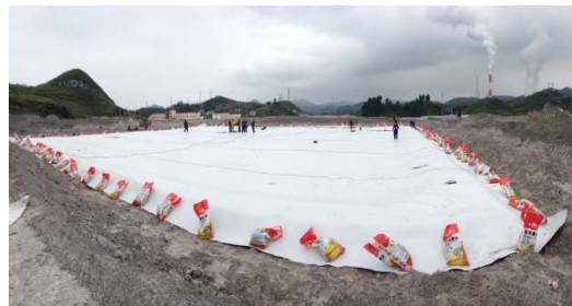
Fig. 9 Installed White Leak Location Liner.
