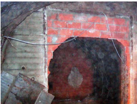
Fig. 12 Masonry wall after explosion [2].
