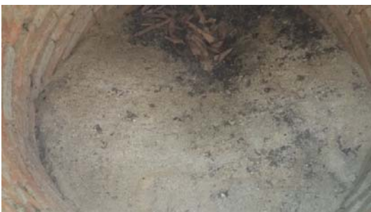
Figure 8 Sand injected into wells of several houses replacing the groundwater.
