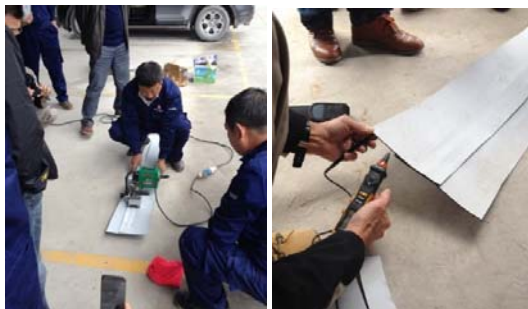
Fig. 7 Trial welding via Iso-wedge welder (left) and check conductivity at weld flap (right).
