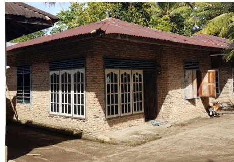
Fig. 2 Unreinforced masonry building
