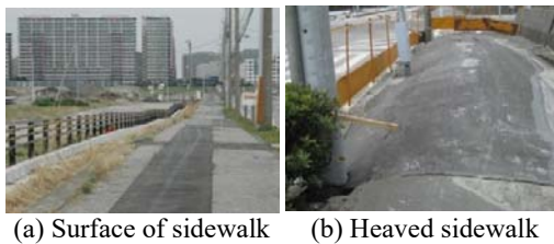
Photo 1 Uneven settlement near the observed sites
