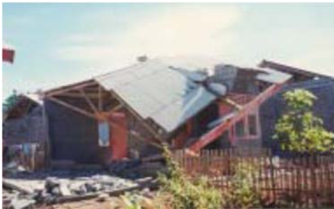
Fig.1 The collapsed building of unreinforced masonry building [2]
