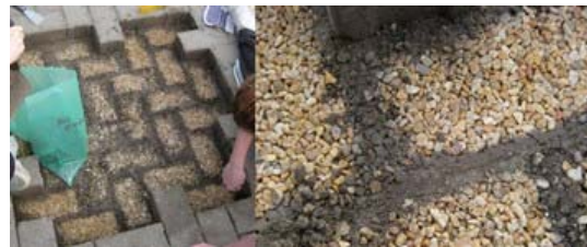
Fig. 2. Sediment Accumulation Pattern on Bedding Aggregate [2]
