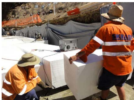
Fig. 3 Showing placement of EPS blocks
