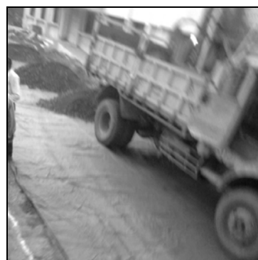
b) GSB spreading on Geotextile
