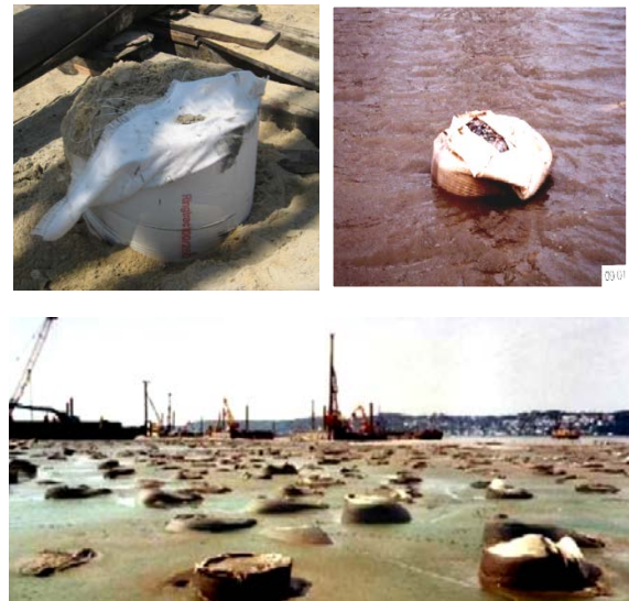
Fig. 8 Examples of completed GECs: in a sand platform, in streaming water, in sludge.
