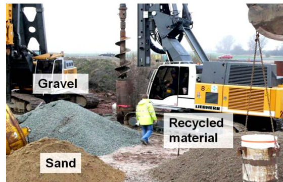
Fig. 5 Different fills for GEC in a field trial.
