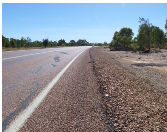
Fig. 2 Cracks on the roadway sealed with bitumen.
