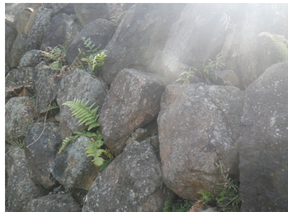
Fig. 1 Masonry revetment and some plants colonizing the spaces between stones.
