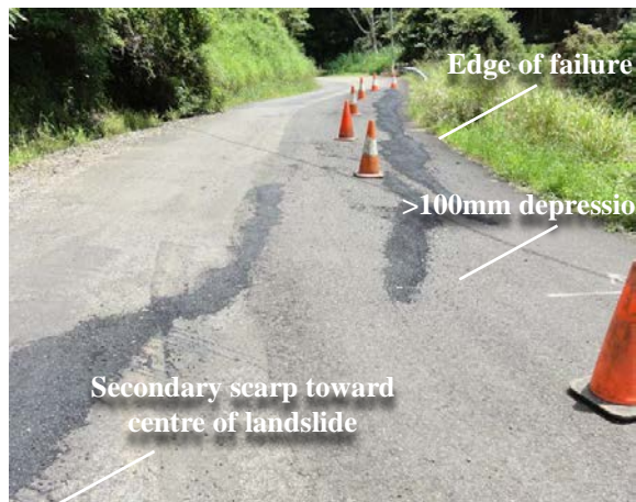
Fig. 1 Areas of subsidence and tension cracks
