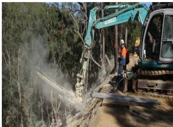
Fig. 5 Drilling of soil nails
