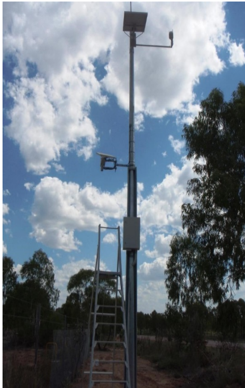
Fig. 5 Completed installation showing logger box (bottom), satellite antenna (mid), weather station and solar panel (top).
