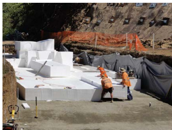
Fig. 3 Showing placement of EPS blocks
