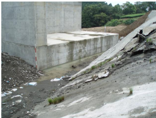
Photo 3 Damage to Temporary Slope Mitigation Works Prior to Permanent Works
