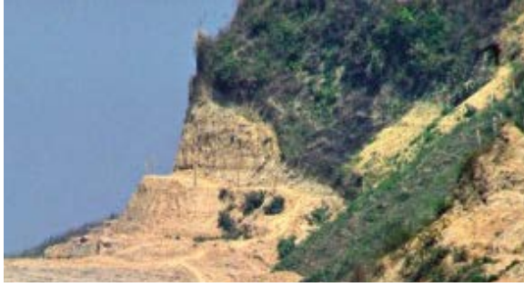
Fig.4 Natural slope was illegally cut to stiffer inclination susceptible to failure (source: Daily star)
