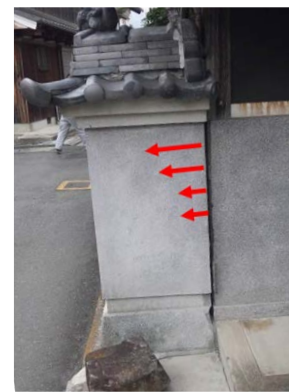
Fig. 2 Inclined fence of a house at B1
