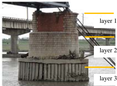
Fig. 1 An existed pier in the water way with temporally reinforced by micro-piles
