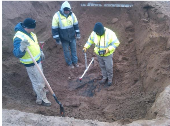
Fig. 7 Photo of excavation near leak signal and pin-pointing the leak
