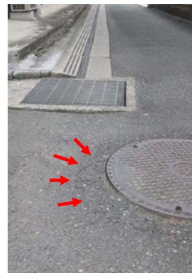
Fig. 1 Subsidence around a manhole at B1
