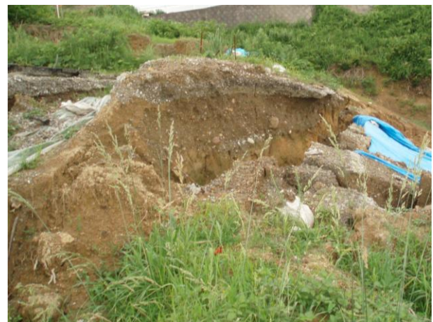
Photo 2 Slope Failure Triggered by Excavation
