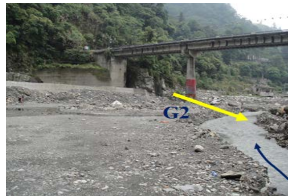
Fig. 3 ERT inspecting a bridge shallow foundation.
