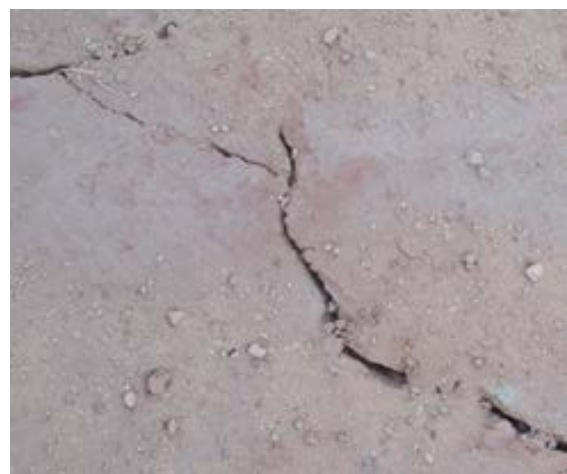
Fig.2 Typical ground cracks reported in shale formation.
