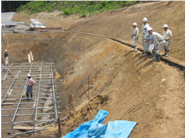
Photo 4 Erosion occurring on 1:1.0 (V:H) Temporary Cut Slope
