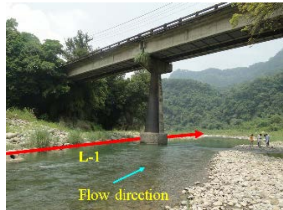
Fig. 6 ERT inspecting a bridge caisson.
