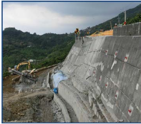
Fig.7 This shows the retaining wall damaged by deep sliding when Morakot happened in 2009.
