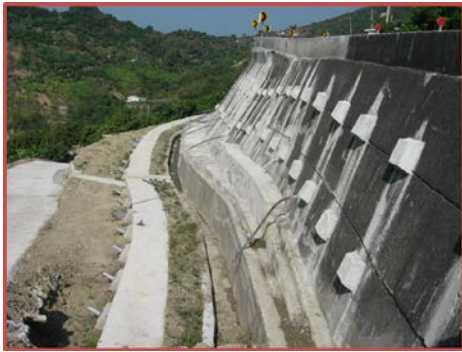
Fig.8 This shows the reinforced retaining wall.
