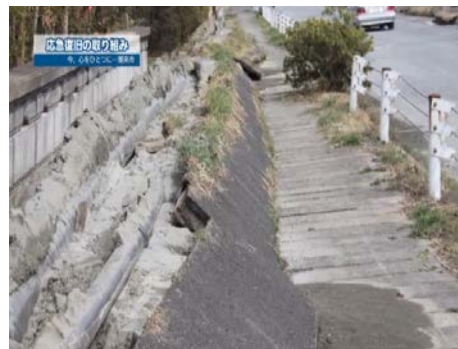
Fig. 1 Damage as floating of underground structure due to liquefaction
