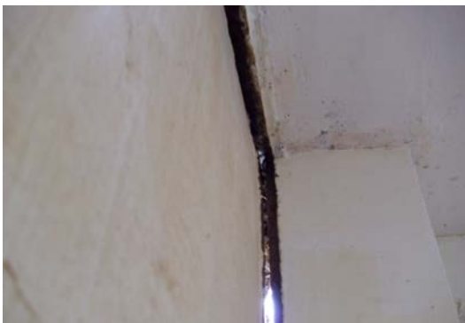
Figure 2. Opening at expansion joint.
