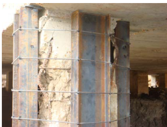
Figure 4. One of buckled basement columns
