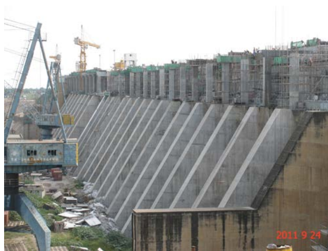
Fig. 2: Thickening and Strengthening of buttresses
