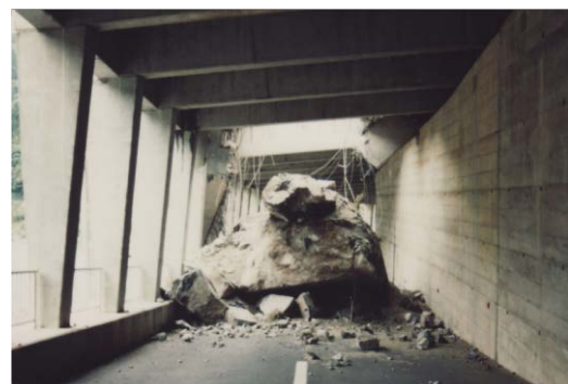
Fig. 3 Failed rockshed by large rockfall
