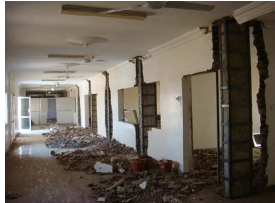
Figure 7. Metal jacketing of second floor columns
