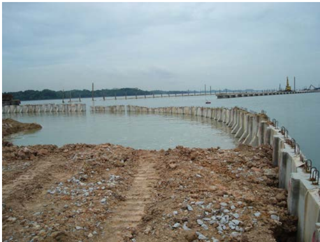
Fig. 5 Conditions of failed quay wall.
