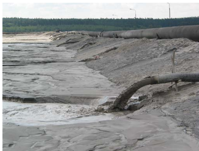
Fig. 2. Observed plunge pool at discharge point at the Żelazny Most dump [3].
