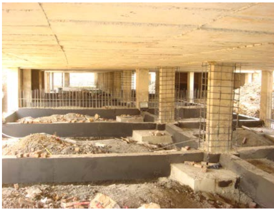
Figure 6. Modification of foundation and concrete jacketing of short columns
