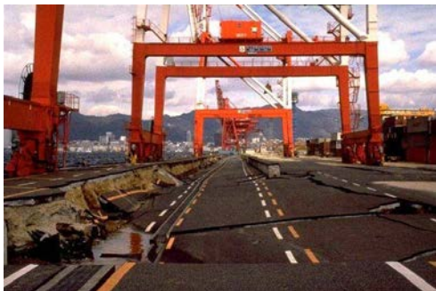
Fig 2 : Liquefaction damage
