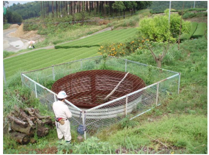
Photo 6 Drainage Well in Tea Plantation Field
