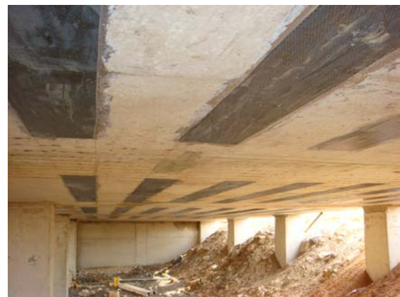
Figure 8. CFRP for basement cover slabs
