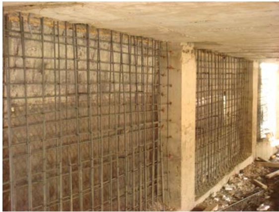
Figure 9. Installation of shear walls at expansion joints
