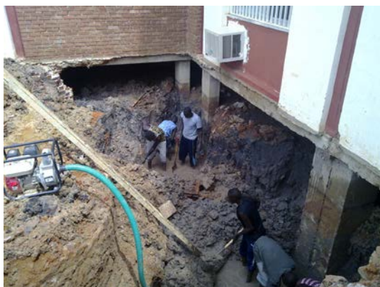
Figure 3. Dewatering during excavation.
