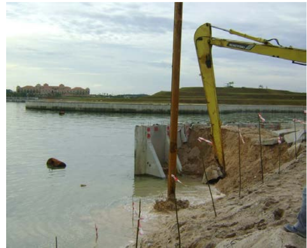
Fig. 8 Stone column installation work at site
