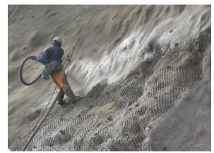
Fig. 7 A part of completed composite for slope protection (Sasagatake mountain, Iga city, Mie)
