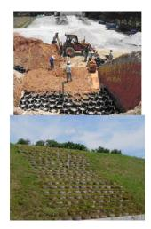
Figure 16 Constructing the trial scrap tire wall
