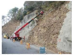
Fig. 2 Cutting of trees and cleaning of the slope before pacing the mesh (Sasagatake mountain, Iga city, Mie)
