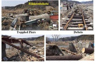
Fallen Girders Scoured embankments Figure 14: Damage to railways and railway bridges
