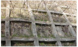
Fig. 11 Completed composite frame with horizontal joints for earth slope protection (Sasagatake mountain, Iga city, Mie)
