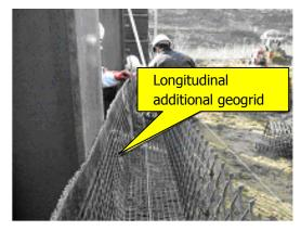
Fig. 10. Installing of longitudinal additional geogrid.
