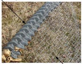
Expanded mesh in spread from \_\_\_\_\_ Fig. 1 Mesh used for composite technology for slope protection
