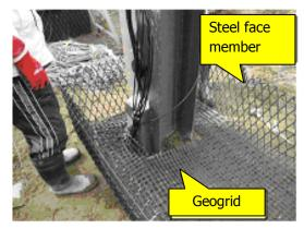
Fug. 8. Installing of steel face member and geogrid.
