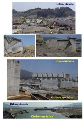
Figure 15: Views of damage to roadways and roadway bridges.
