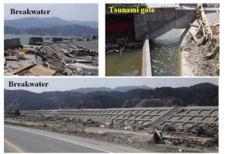
Figure 8: Views of the state of counter-measures after the tsunami.
