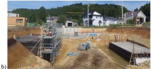
Fig. 27 The first GRS integral bridge for the new bullet train line at Kikonai between Shin-Aomori and Shin-Hakodate stations: a) overall dimensions; and b) a picture at the end of August 2011 (by the courtesy of Mr. Yamada, Y.).
