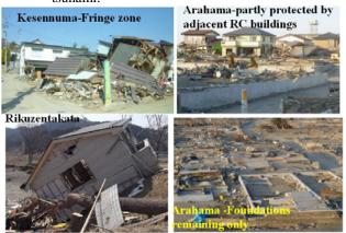
Figure 9: Views of damage to timber buildings.
