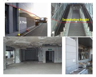
Figure 16: Views of damage to Sendai Airport
