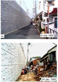
Fig. 11. GRS RW having a FHR facing at Tanata; a) immediately after construction & a typical cross-section; and b) one week after the 1995 Kobe Earthquake (Tatsuoka et al., 1997, 1998).
