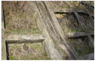
Fig.9 Completed composite frame with vertical joint for slope protection (Sasagatake mountain, Iga city, Mie)
