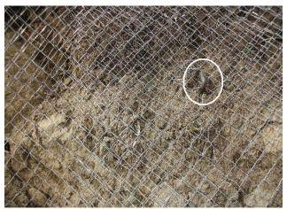
Fig. 4 Anchored pin for fixing the mesh on the slope
