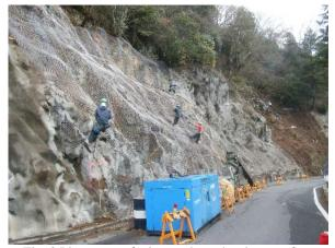
Fig. 3 Placement of wire mesh on the slope surface (Sasagatake mountain, Iga city, Mie)
