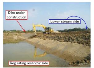
Fig. 15. Dike of the regulating reservoir during construction
